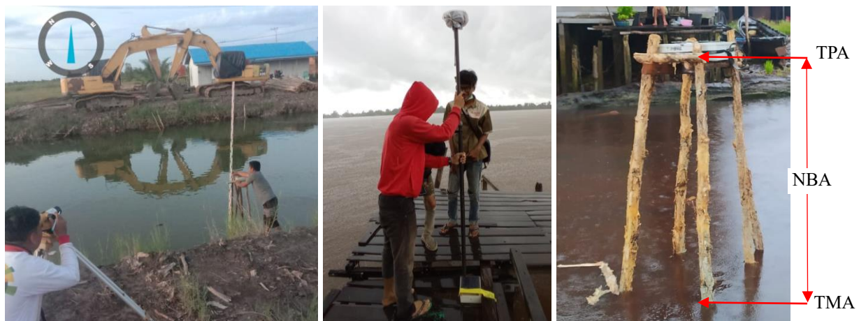
Figure 2. Elevation measurement and installation of AWLR tools and illustration to determine NBA
